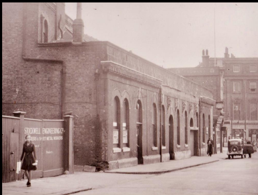
Greenwich Park Station before its demolition. No. 7 would have been just to the right of the Gate.
